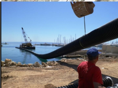
-project SPLIT port sea outfall ID 1200
